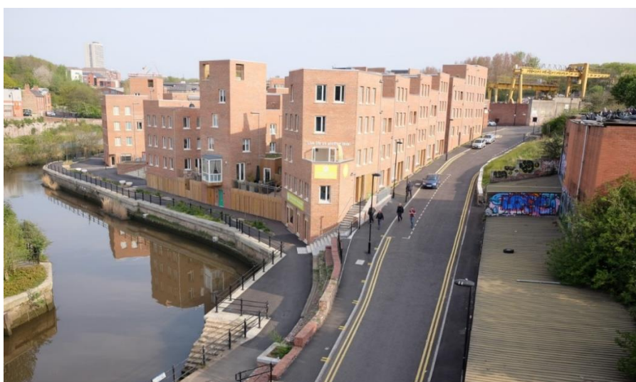
Figure 2.3: The Malings, Newcastle-upon-Tyne, updates the traditional 'Tyneside flat' typology in a contemporary style whilst also responding to the riverside context – all homes benefit from a river view.
