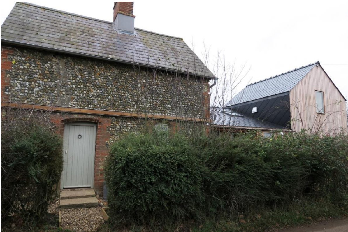
Figure 2.8: Contemporary extension in Norfolk using modern construction methods but drawing design influences from the historic dwelling such as roof line, building height and form.
