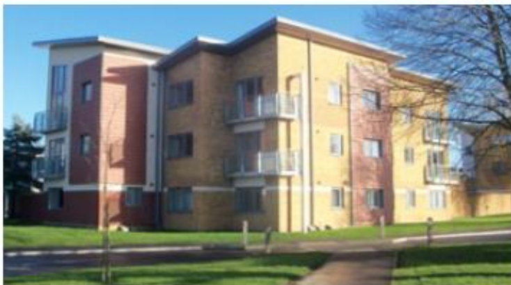
Fig 3.15: The North Loose Neighbourhood Development Plan 2015-2031 (made in May 2013) included images of developments they do not think reflect local character.
